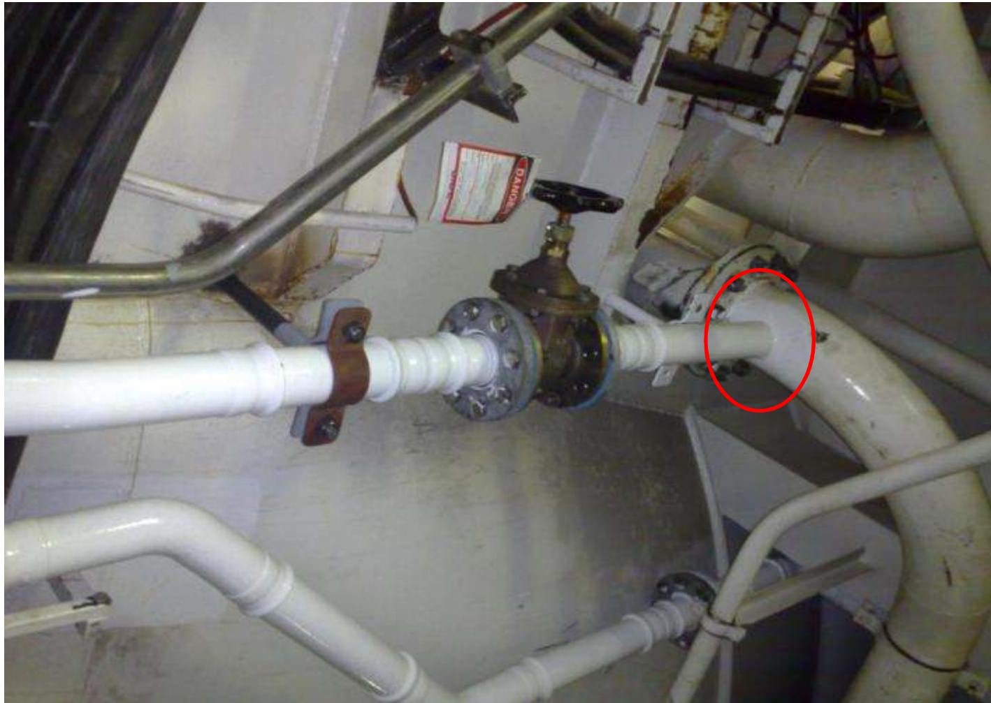
90/10 Copper Nickel Press Fit System coming off Existing Fire Main from a Welded Spigot - HMAS Manoora
